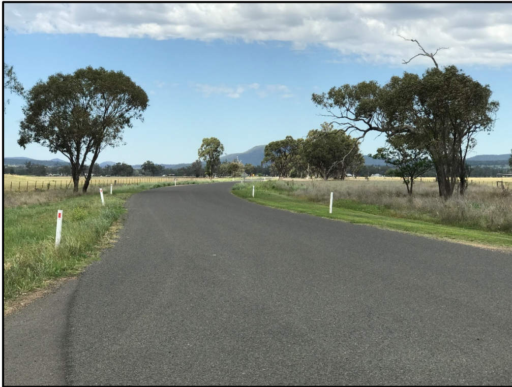
Photo 3 – Typical cross section for Kelvin Road to the south of Orange Grove Road
