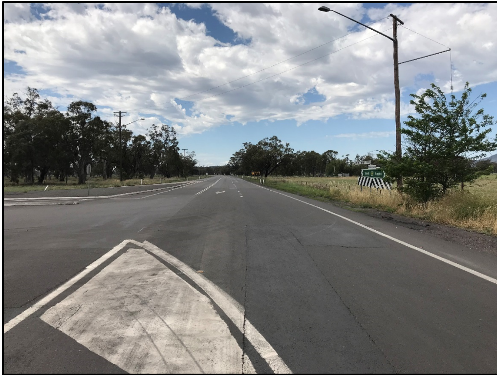
Photo 7 – View east along the Kamilaroi Highway showing sheltered right turn lane for vehicles turning into Blue Vale Road
