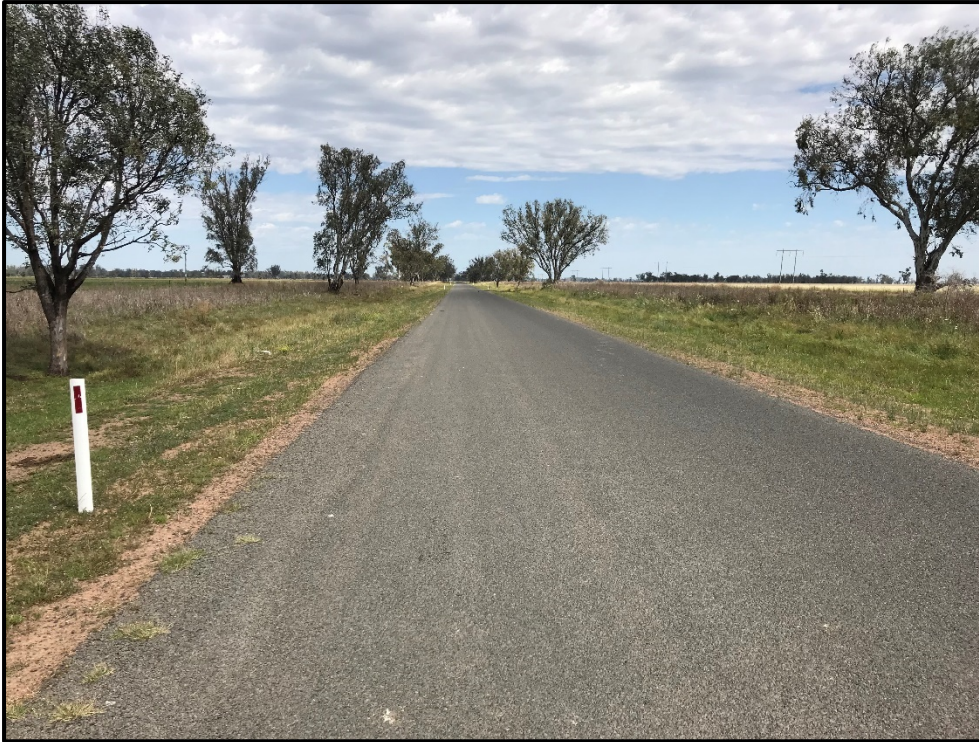
Photo 2 – View along Orange Grove Road to the west of the subject site where the road has a sealed pavement and edge marker posts
