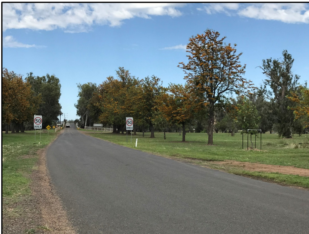
Photo 4 – Section of Chandos Street to the immediate north of the Namoi River bridge. Note 50 km/h urban area speed limit is located here.
